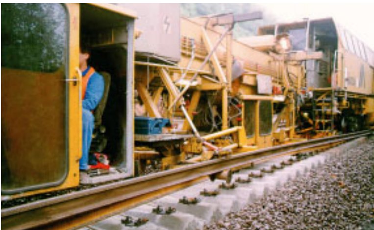
Automated installation of the wide sleepers
