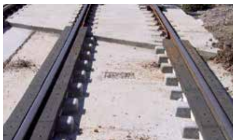
Concreted track with green track chamber elements and level crossing
