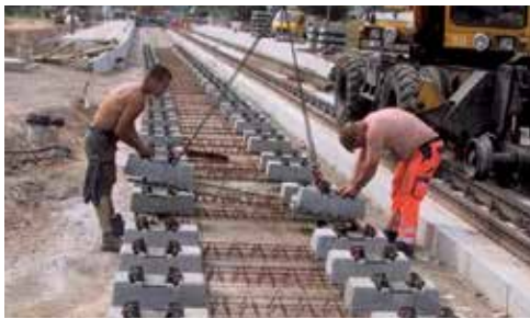
Positioning of the bi-block sleepers
