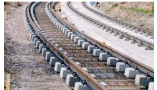
Completely assembled and aligned track panels
