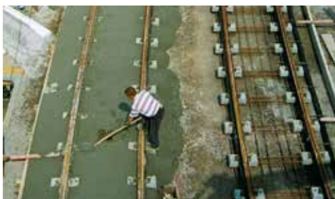
Concreting of the track panels
