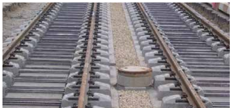
Installed and properly aligned track panels
