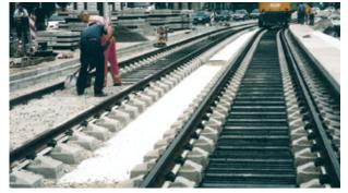
**GREEN LIGHT FOR THE TRAMWAY** Both the ATD-G and the RHEDA CITY GREEN models can be installed with conventional equipment for street and track construction. The small number of working steps in laying the track enable fast construction work.
