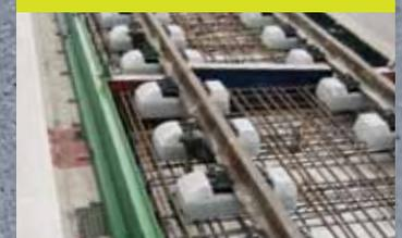
more than  $\pm 2$  mm with reference to each other – dimensions that demand a maximum of exactness in concrete construction. The top-down installation procedure inherent to this system can optimally satisfy these exacting requirements. Production of special sleepers by RAIL.ONE – with manufacture and installation of the RHEDA 2000® system by local construction companies – allows optimal economical cost/benefit relationship: both for RAIL.ONE as well as for the local industry.
