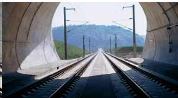
**The flexible way for all applications** The RHEDA 2000® ballastless track system is ideal for applications on embankments, on bridges, in tunnels, as well as for turnouts and with vibration-optimized mass-spring systems. Installation of noise absorbers attenuates noise from wheel-rail rolling and vehicle power-plant operation.
