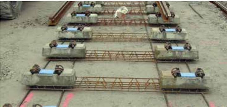
Adjustment and fixing of the track panel, laid out onto the subgrade, in proper direction and height
