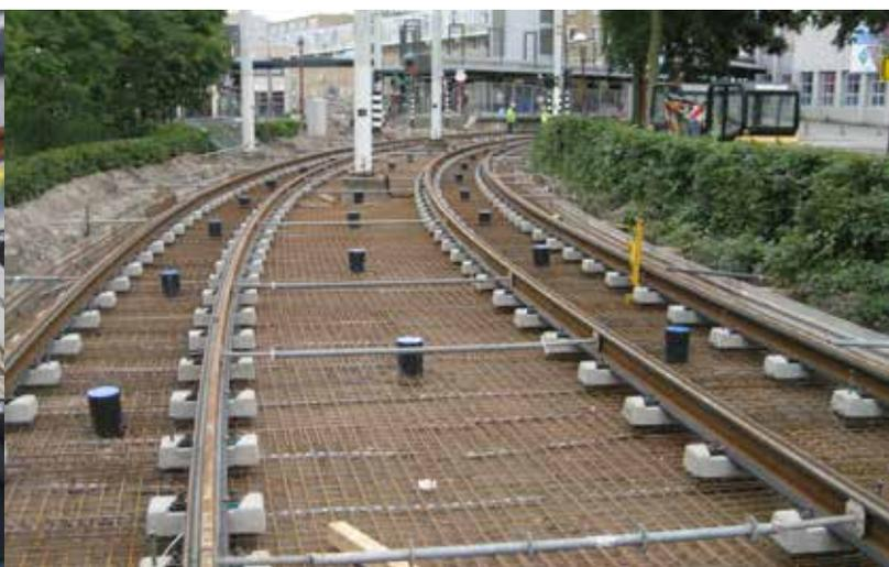
**UTRECHT, NETHERLANDS** The tram operator BRU realized in 2012 an upgrade project of the existing SUNIJ-Lijn in the urban area of Nieuwegein to optimize the track quality. RAIL.ONE supplied for this project the RHEDA CITY system and delivered approx. 820 meters of RHEDA CITY track. In addition, RAIL.ONE supplied turnout bearers for the switches and crossings.
