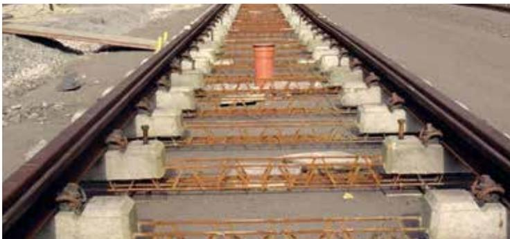
Installation of the sleeper-crib intermediate layer
