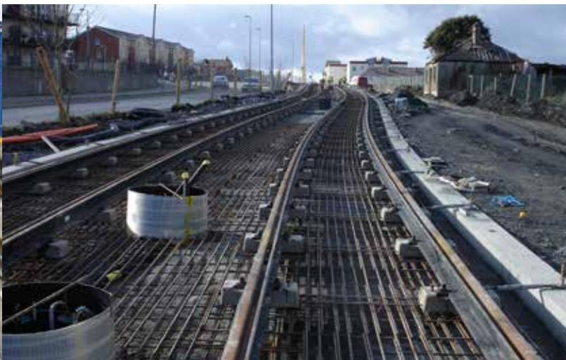
**DUBLIN, IRELAND** In the City of Dublin the RHEDA CITY system has been installed for extension of its tram network on the Dublin LUAS A1 Line, for Sections 401 and 402. For this project, RAIL.ONE delivered about 7,000 RHEDA CITY bi-block sleepers for approx. 5.6 km of covered track and 2.5 km of open track, with delivery to the Dutch construction company BAM Ireland. RAIL.ONE likewise supplied turnout sleepers for the planned tram turnouts.
