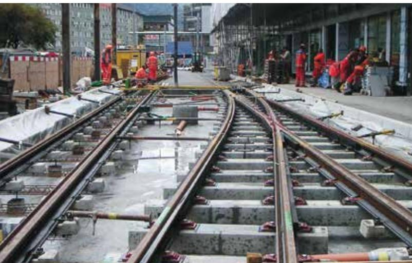
**CHUR, SWITZERLAND** The train station in Chur is the hub of local public transport. As part of alterations of the station forecourt, the tracks of the Chur-Arosa line were relocated. The RHEDA CITY ballastless track system was then installed there, for the first time in Switzerland. In addition to delivery of the main-track and turnout sleepers, RAIL.ONE was also responsible for system supervision of track installation.
