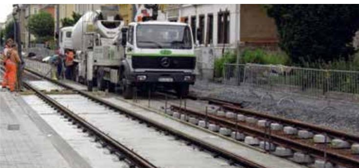
Installation of chamber elements in the spaces between the rail head and the rail flanges
