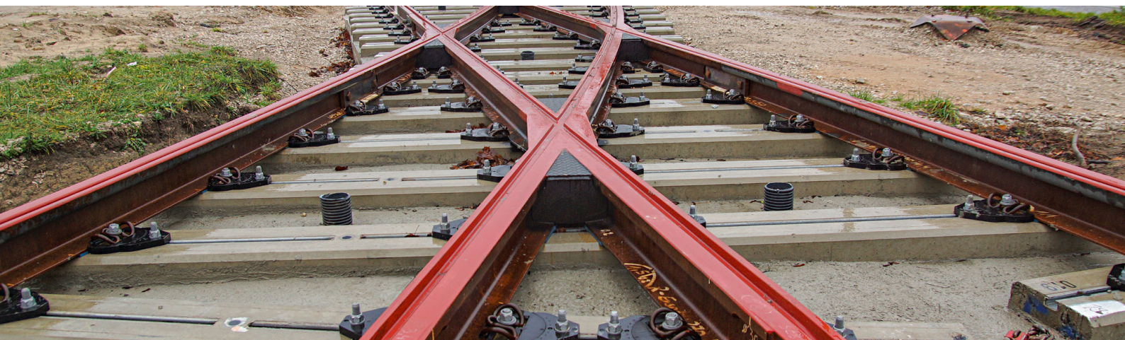
Crossing with AS-SKL fastening in installed track
