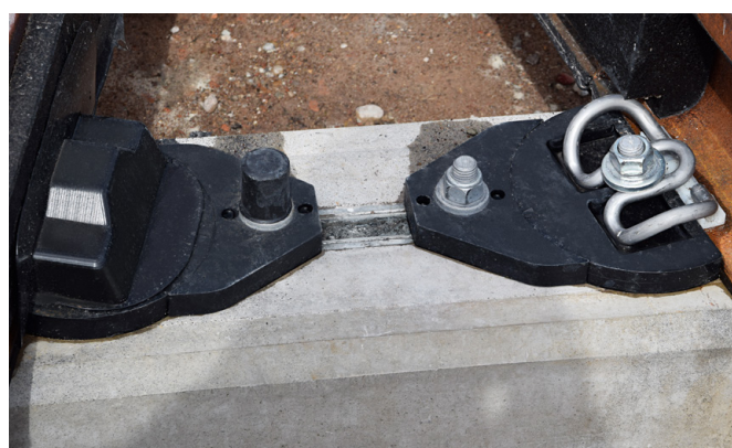
Anchor rail fastening with and without cover cap
