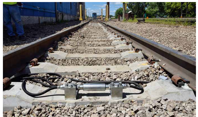
Figure 4: sensors on top of the sleeper center
