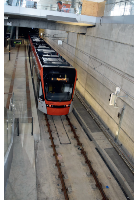
6: Rheda City ballastless track system at the Flesland airport terminal platform Photo: Rail.One
